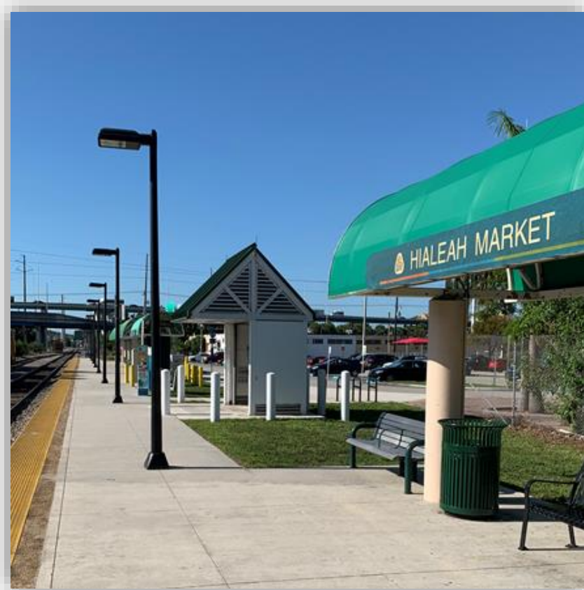
Existing Station – West Side Platform
