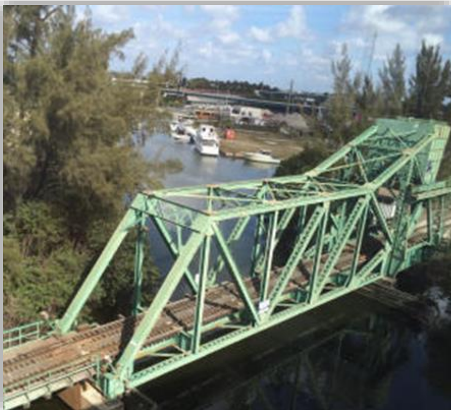
Existing Single Track Bascule Bridge
