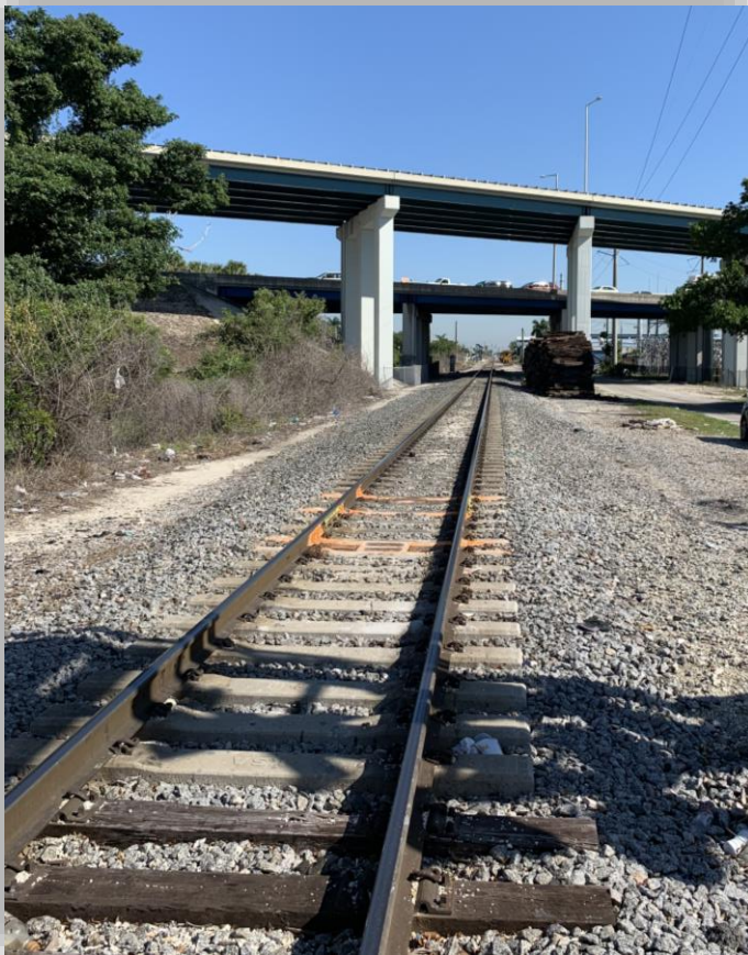
Existing Single Track
